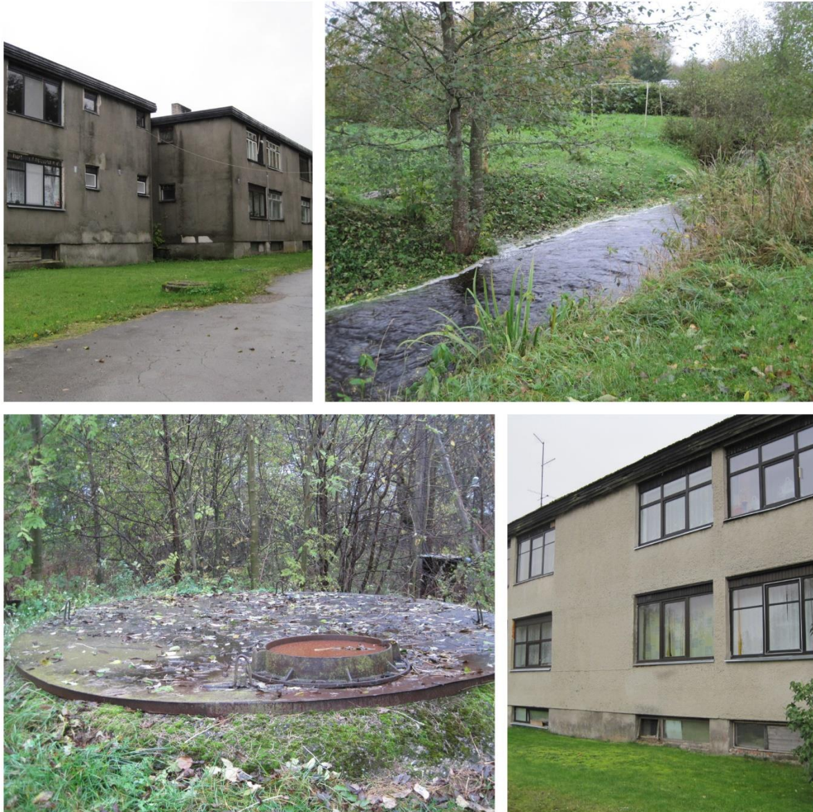
Picture 42. Valkla village pilot before construction of WWTP and renovation of pipelines.
