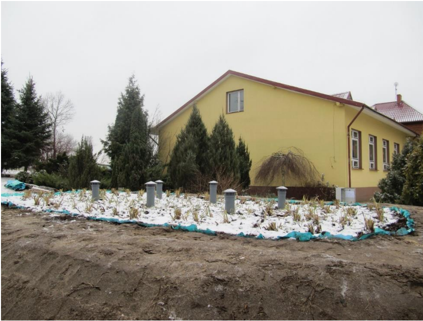
Picture 3. Completed soil filter with vegetation
