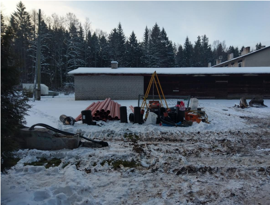
Picture 30. Materials - the building process in Kolgaküla village pilot.
