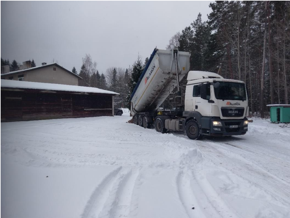
Picture 28. Materials, transportation - the building process in Kolgaküla village pilot.
