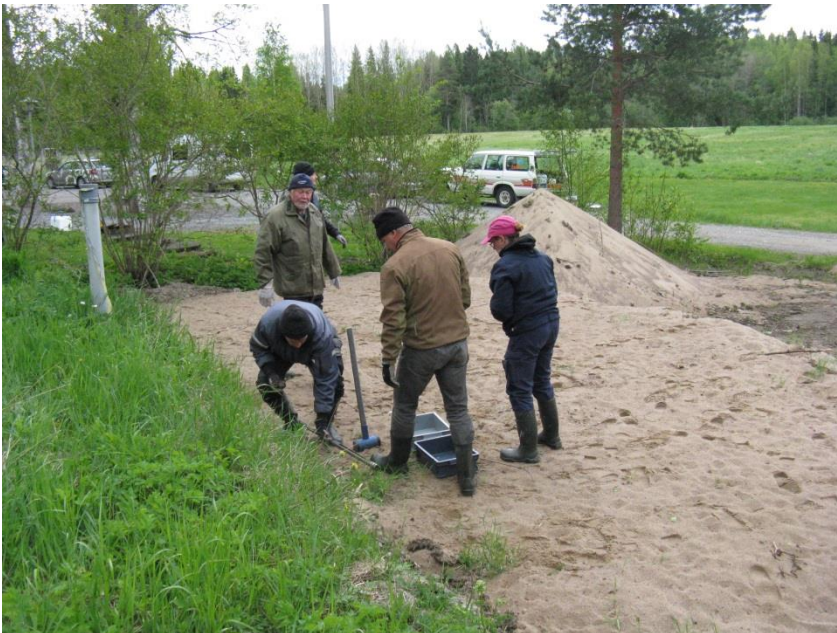
Picture 16. Construction of the Nurmijärvi pilot soil filtration system.
