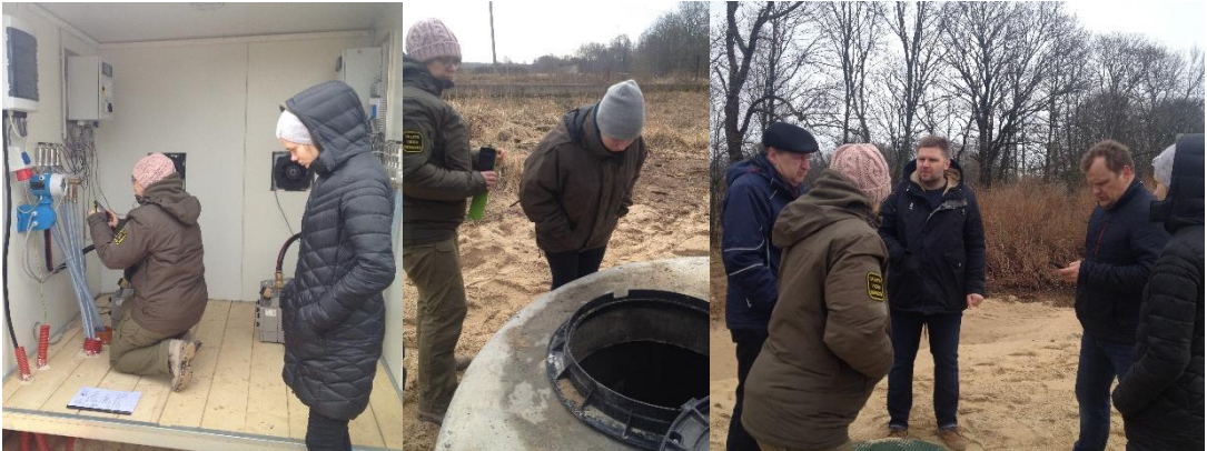
Picture 23. The inspection of WWTP construction carried out by responsible state environmental authority.
