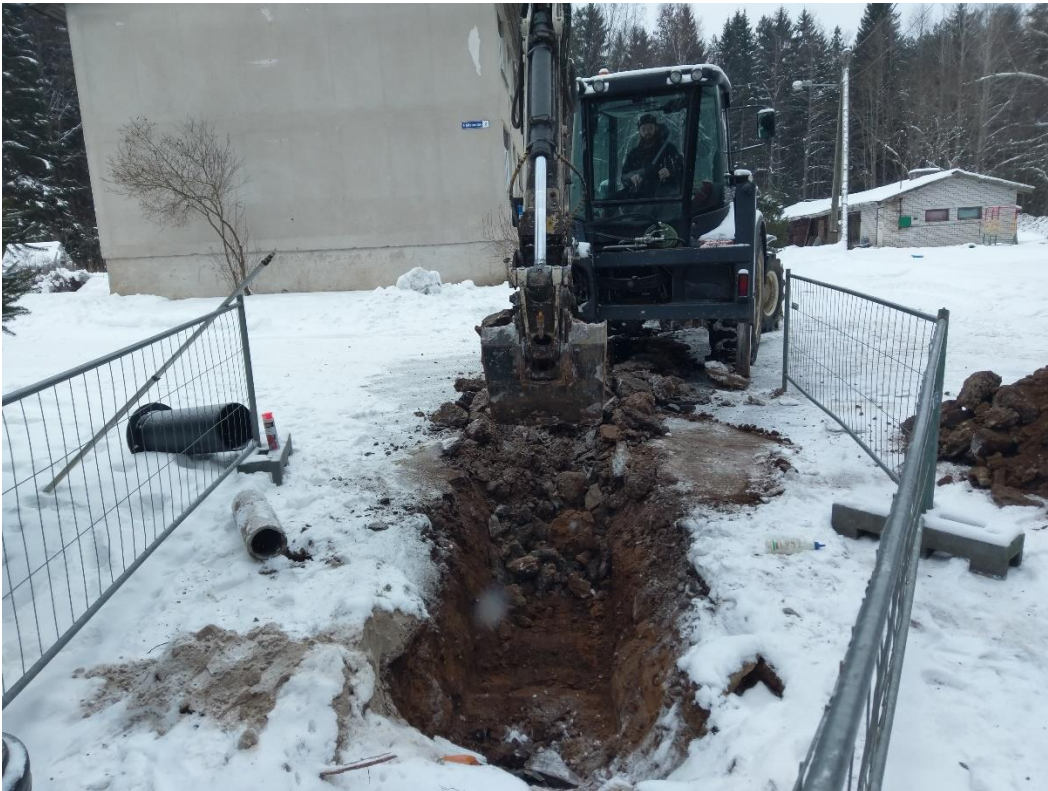
Picture 29. Installation - the building process in Kolgaküla village pilot.
