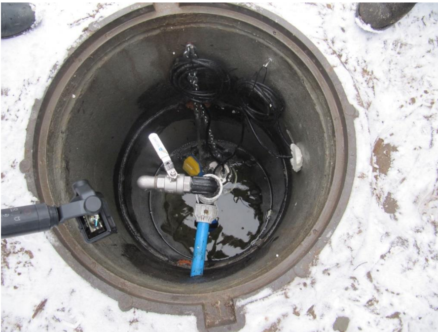
Picture 4. Pumping station
