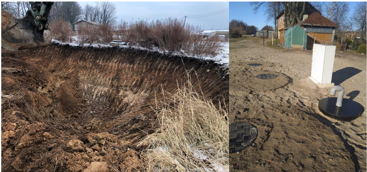
Picture 25. The WWTP during construction.
