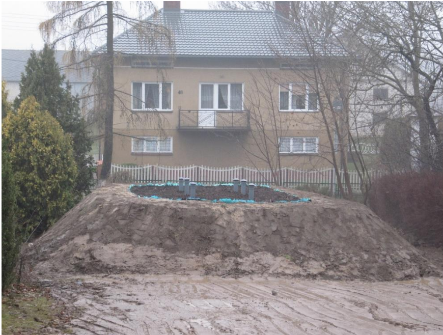
Picture 1. School in Bruszewo with soil filter in building stage.
