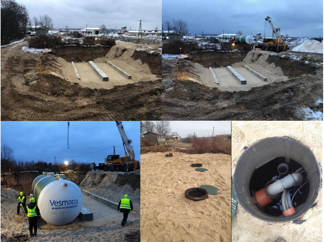
Picture 22. The new WWTP during construction.
