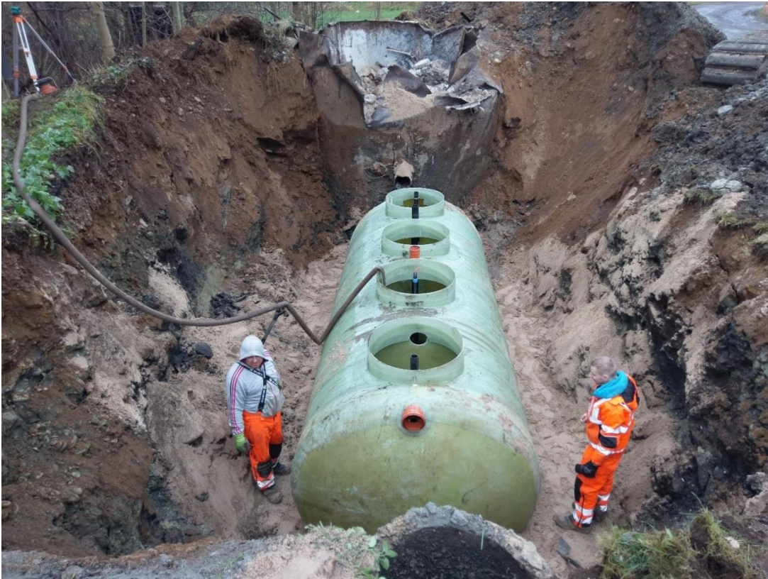
Picture 26. Valkla village – installation of new WWTP.
