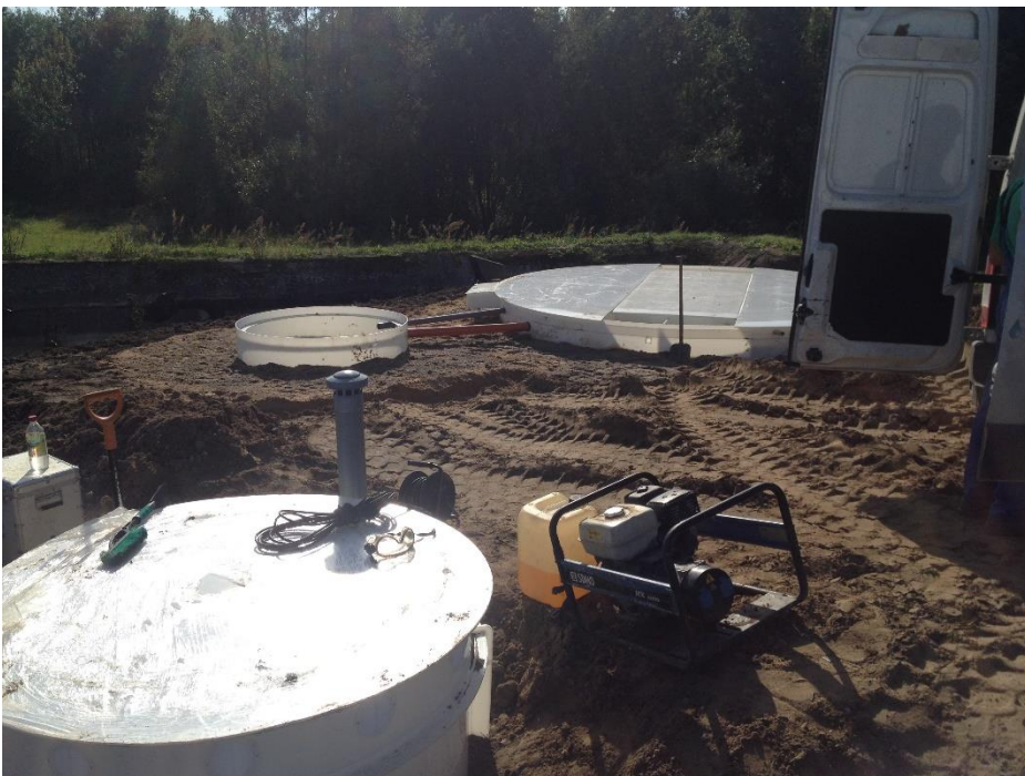
Picture 18. The new wastewater treatment plant during construction
