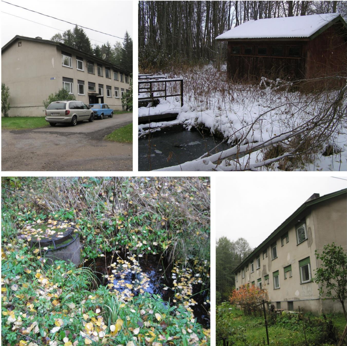
Picture 36. Kolgaküla village pilot before construction.
