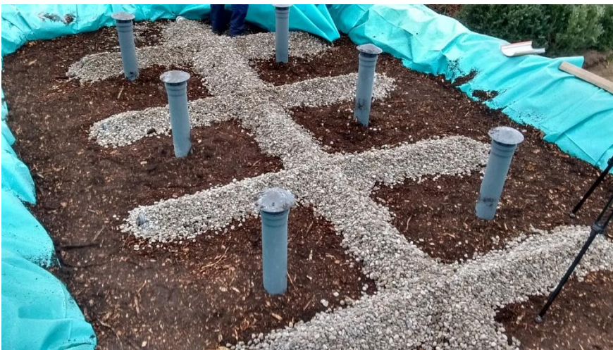
Picture 2. Soil filter with distribution and aeration pipelines before covering
