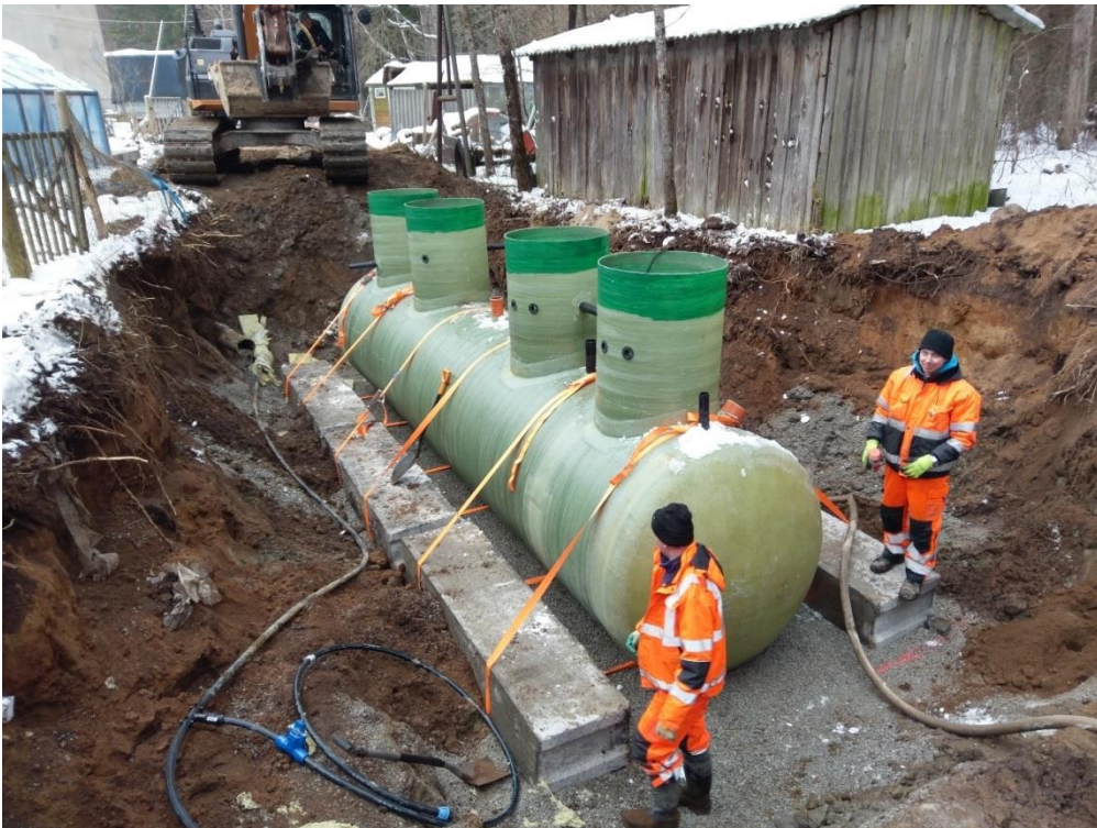
Picture 27. Kolgaküla village – installation of new WWTP.
