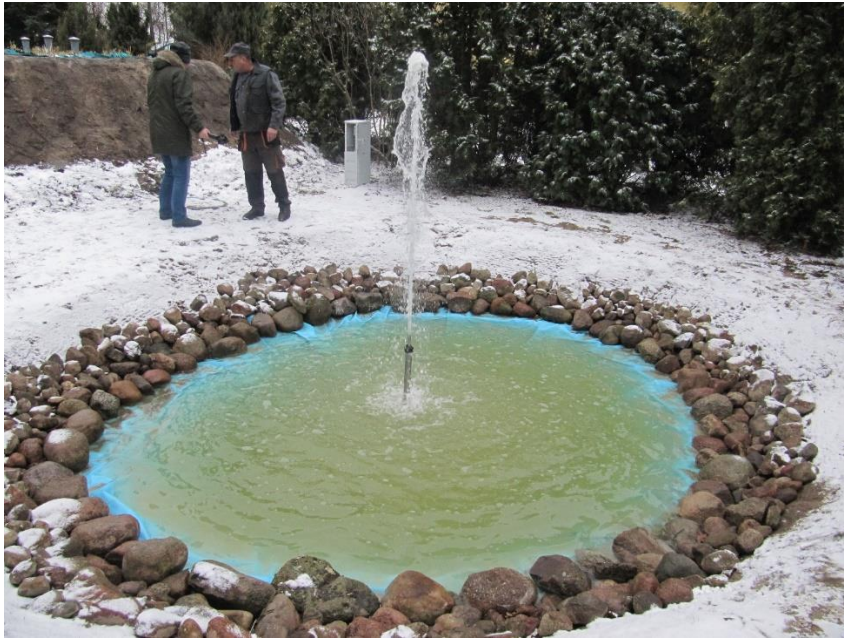
Picture 5. Denitrification pond
