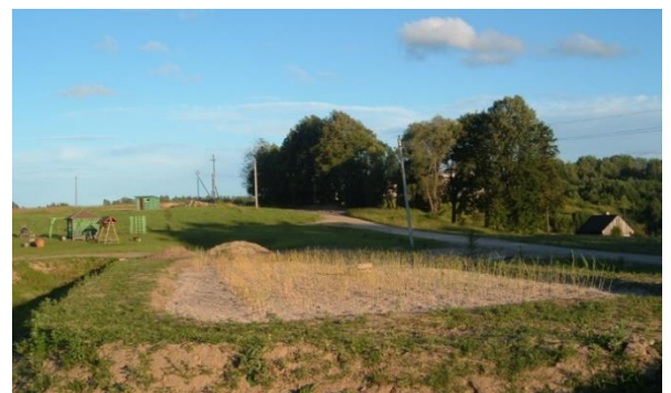
Sub-surface vertical flow constructed wetland
