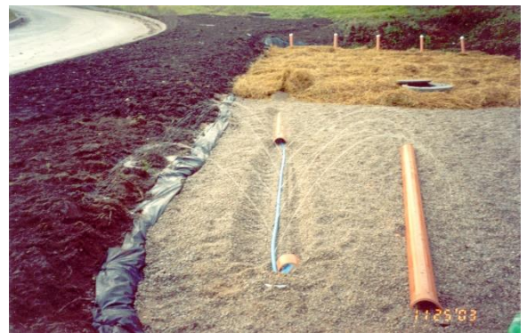
Installation of SSVF CW
