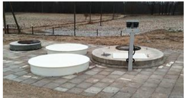
New installation of pre-treatment step
